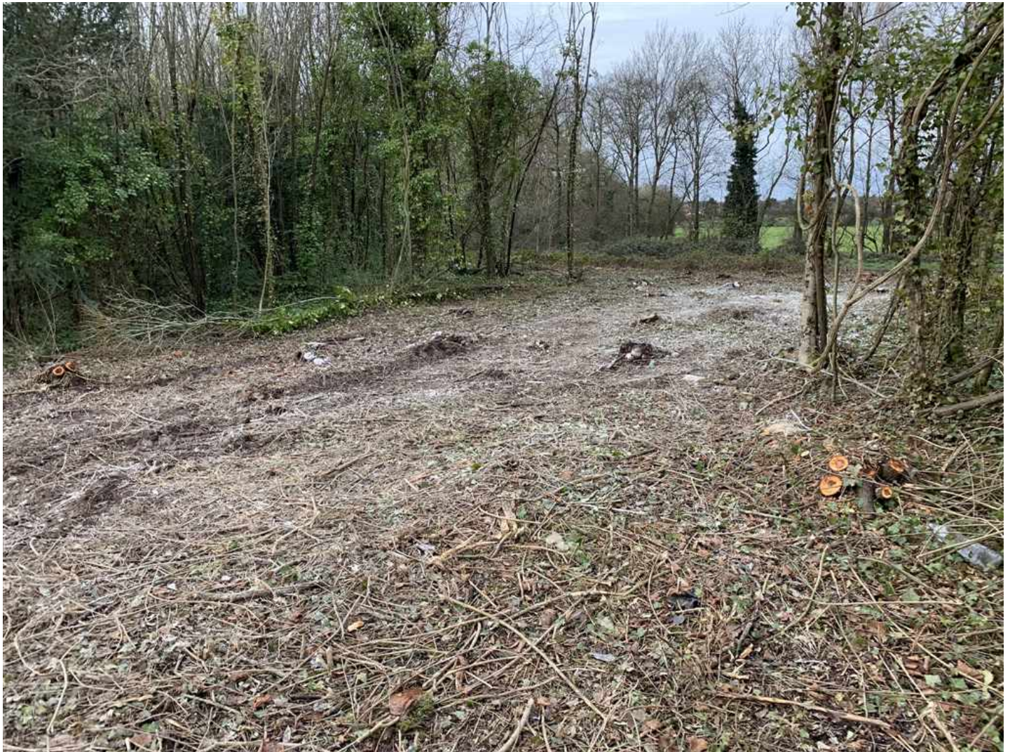
View of devegetation in preparation for drilling BH72405
