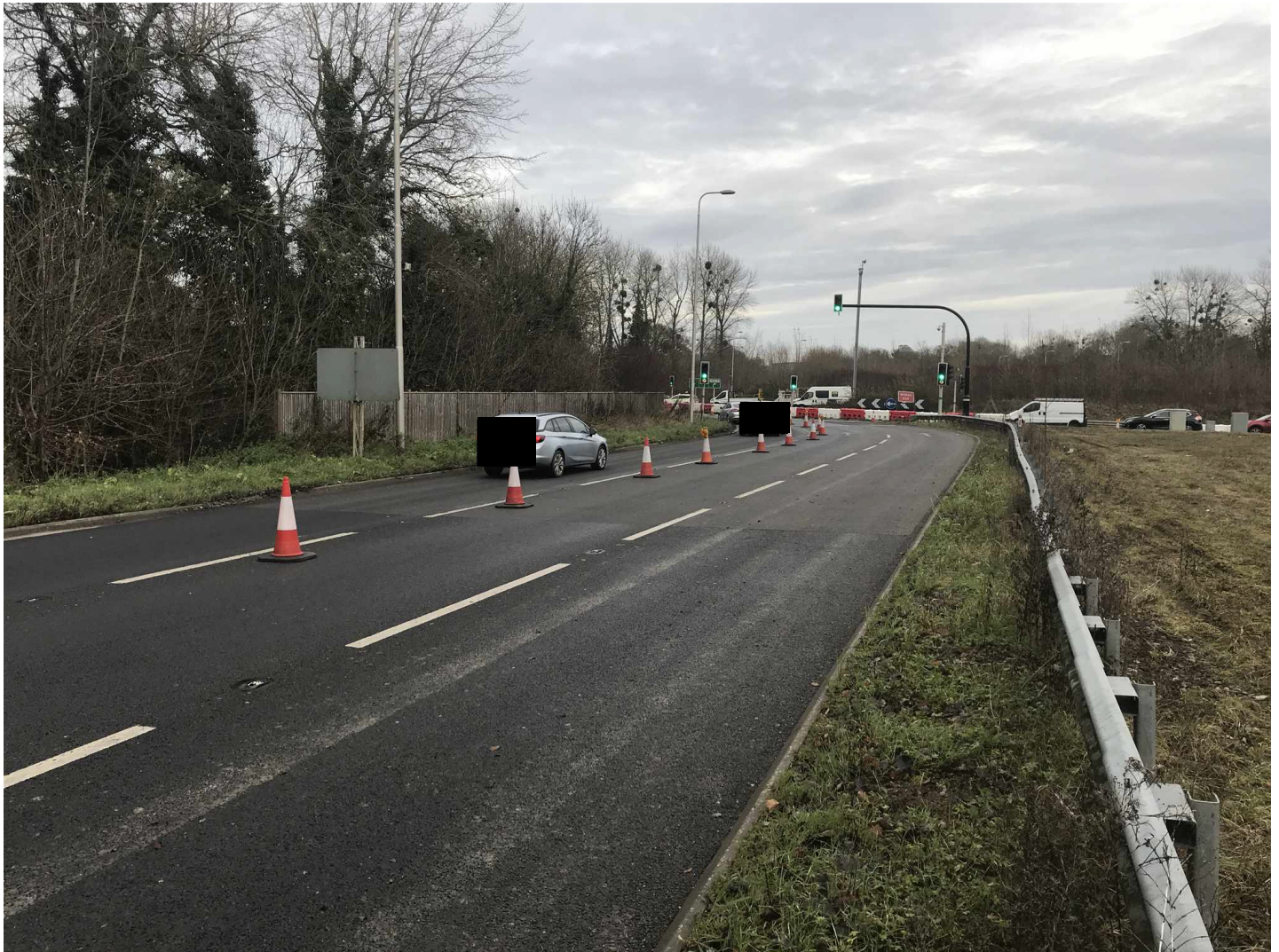
View looking east toward the Countess Roundabout and BH72501
